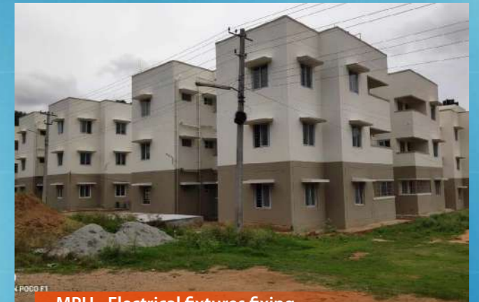
MPH - Electrical fixtures fixing
