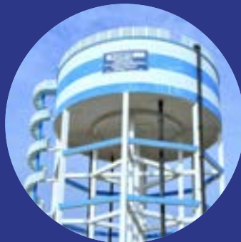
Construction of an elevated water storage facility, supporting reliable water infrastructure through RPP's robust engineering and structural solutions.
