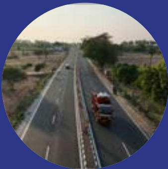
Construction of a road project by RPP, demonstrating its capability in delivering quality highway works with divided carriageways and road safety features.
